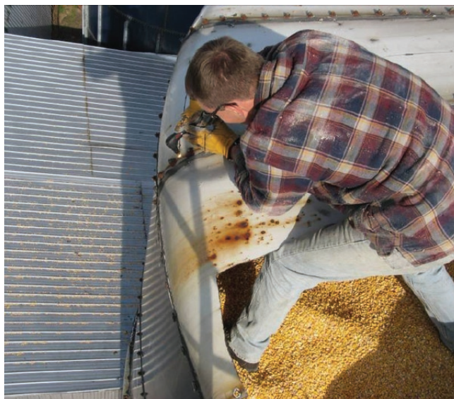
A PLASMA CUTTER IS GOOD FOR SILO REPAIR, INCLUDING GLASS-LINED SILO PANELS.
